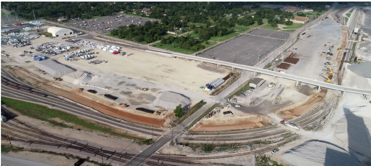
Figure 10: POB - Buford Rail – Eastern End of Project
