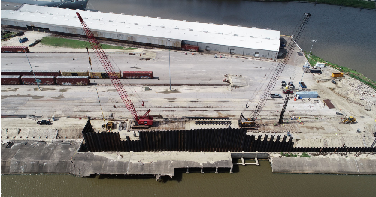
Figure 5: POB – Phase A Construction – New Bulkhead Installation – July 2020
