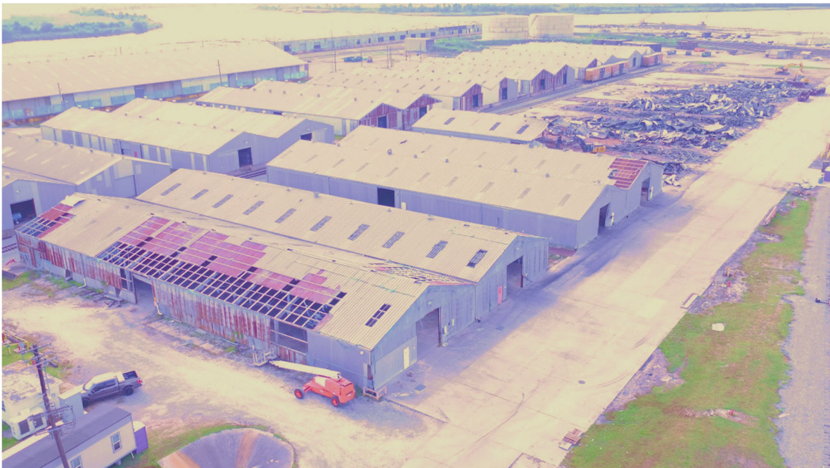
Figure 15: POLC – Demolition of Hurricane Damaged Warehouses in Progress.
