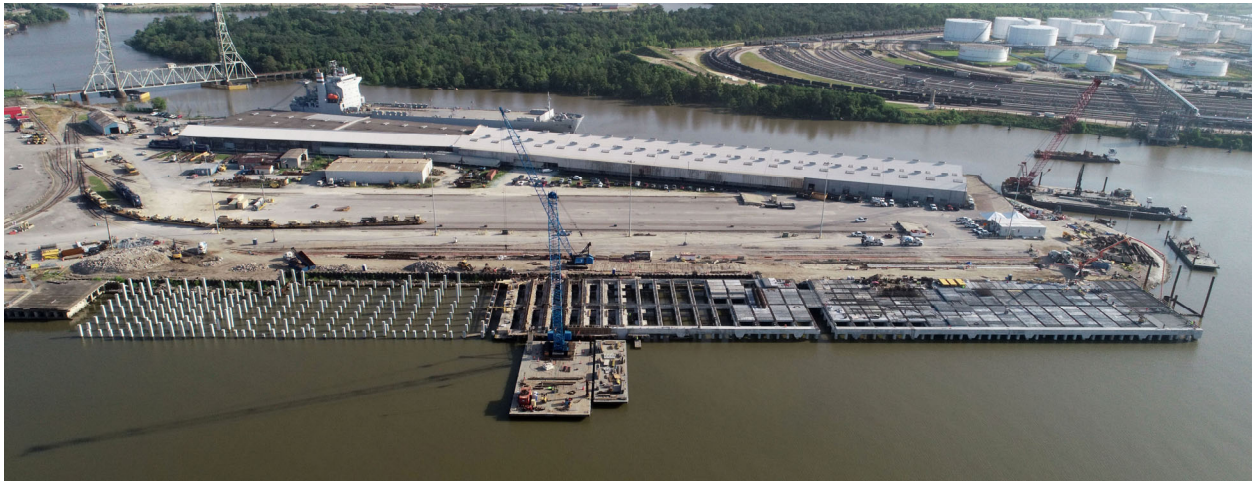
Figure 7: POB – Phase B Construction Progress – July 2023
