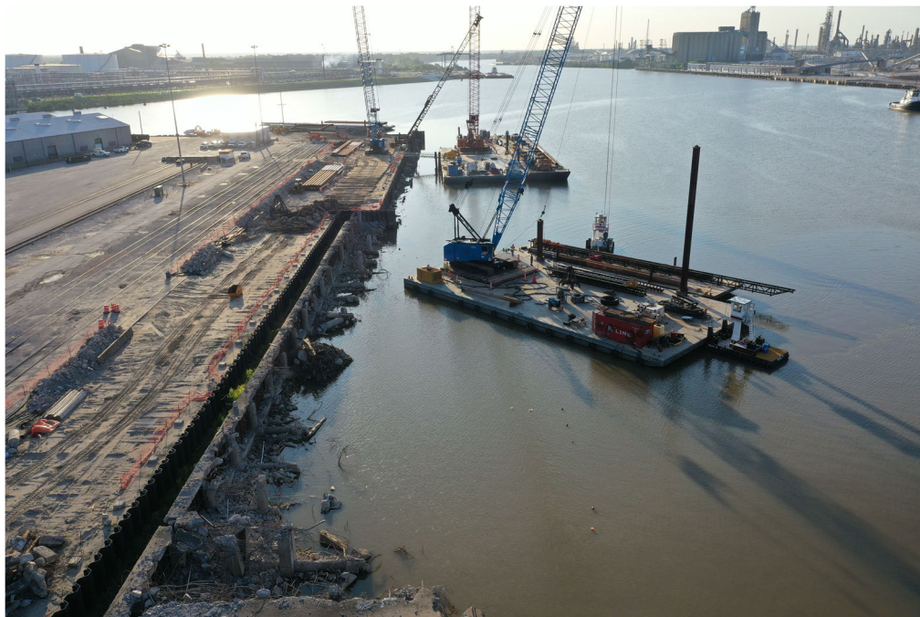
Figure 6: POB – Phase B Demolition – July 2022
