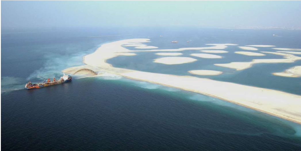
Figure 3- Hydraulic Dredge Filling at Palm Jebel Ali in 2002
