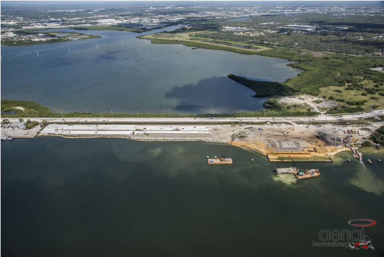
Figure 1- Eighteen (18) Acre land Reclamation Project - Tampa Bay 2015
