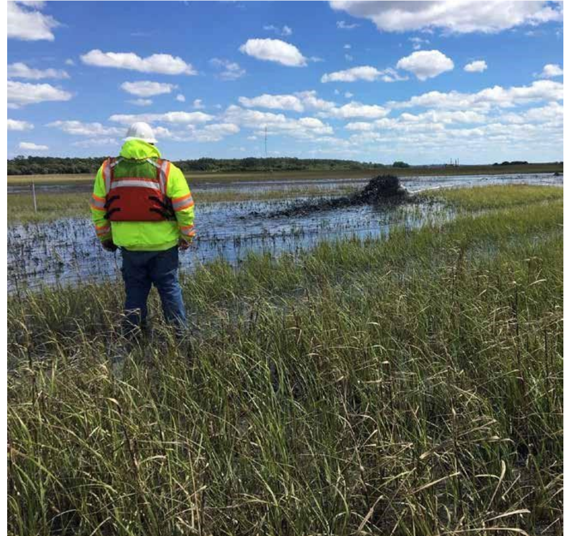
Dredging project manager monitoring dredged sediment placement at the Jekyll Creek Marsh Restoration and Wetland Habitat development Beneficial Use of Dredged Material project, Georgia. (Photo by Clay McCoy, USACE Jacksonville)
