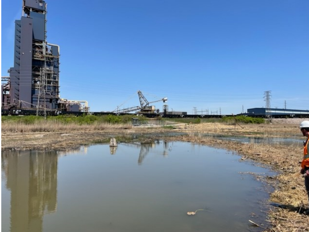
One of the wetlands with the Cleveland Cliffs HBI Facility in the background.
