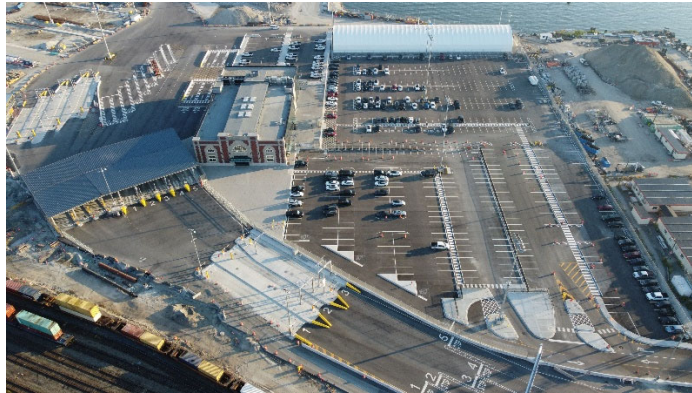
Figure 4: Truck gate completed (July 2022).
