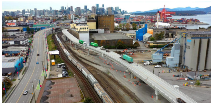
Figure 6: The Centennial Road Overpass being used by Centerm container trucks.
