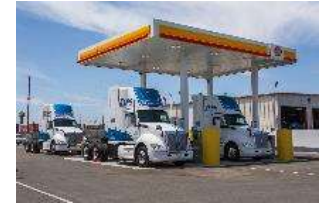
Port of Long Beach Class 8 Drayage Truck H2 Station
